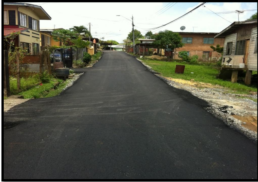
Picture 23: Showing final asphaltic wearing course
