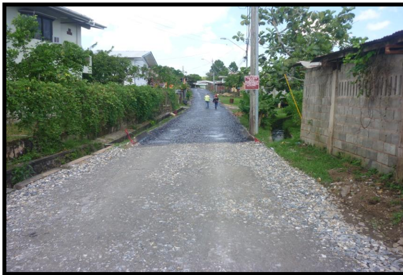
Picture 15: Showing application of prime coat bituminous material along surface prior to paving exercise
