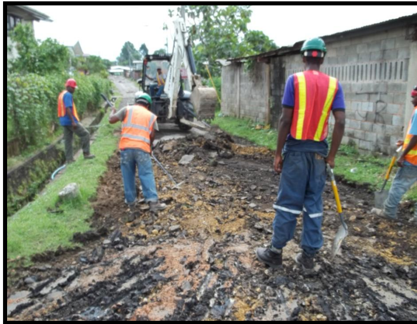
Picture 3: Showing scarifying along roadway
