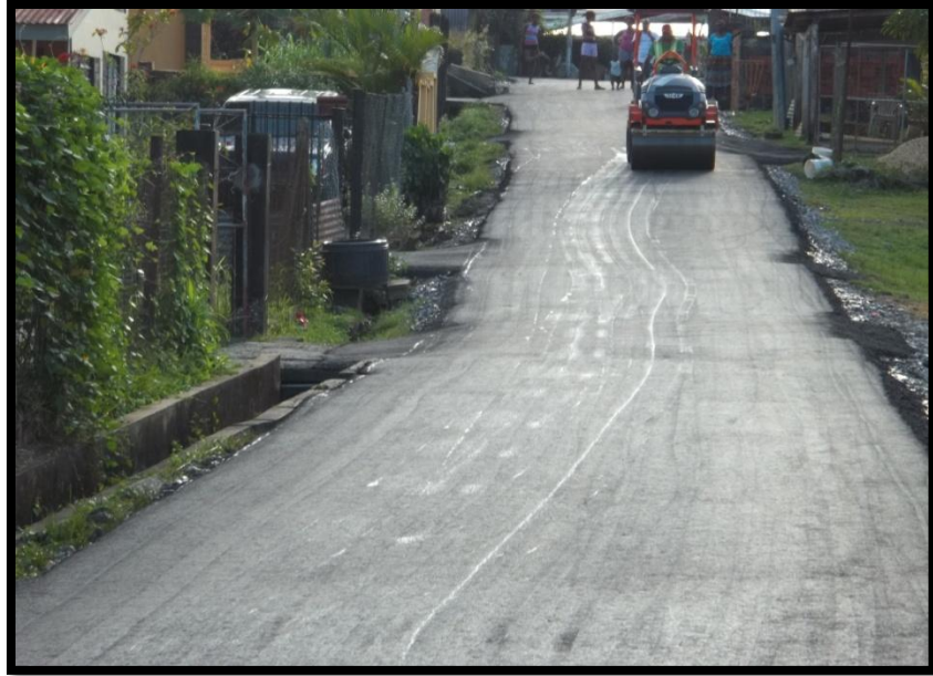
Picture 21: Showing final compaction of asphaltic hot mix using pneumatic roller
