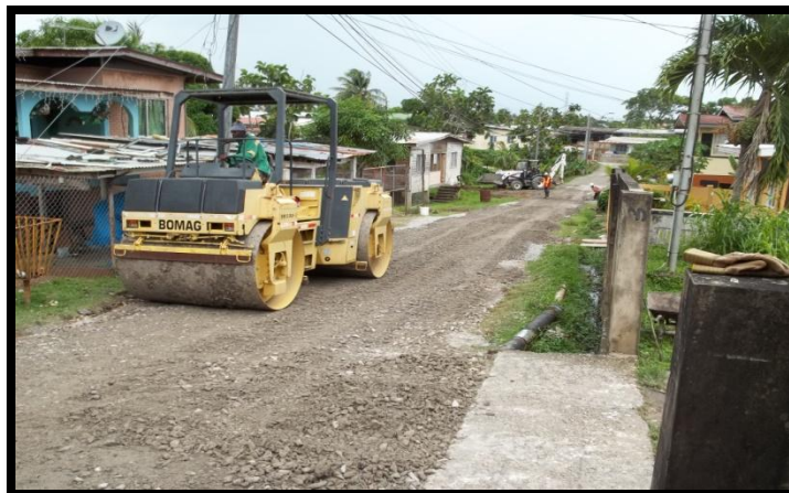
Picture 9: Showing compaction of base course material
