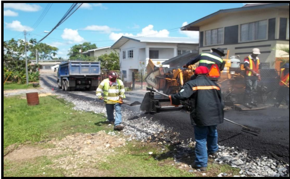
Picture 16: Showing methodology of spreading asphaltic hot mix – including offloading, raking and shovelling
