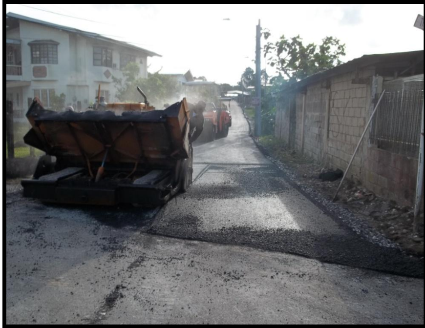
Picture 17: Showing spreading asphaltic hot mix
