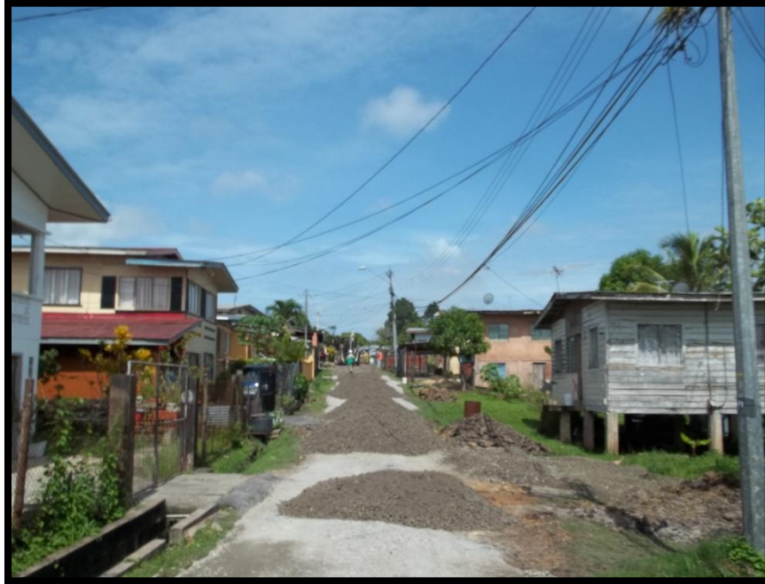
Picture 5: Showing procedure of spreading base course material
