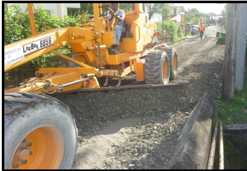
Picture 11: Showing final rectifying of base course level using grader
