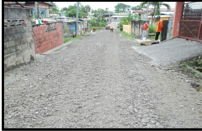
Picture 7: Showing base course material spread along roadway dimensions
