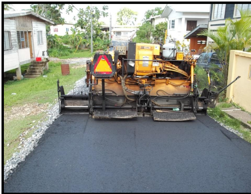
Picture 17: Showing spreading asphaltic hot mix
