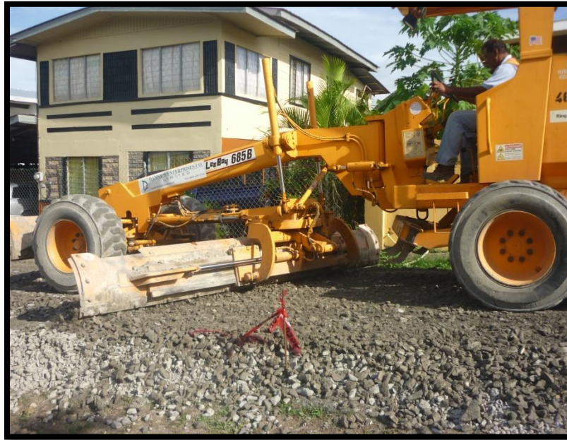
Picture 12: Showing final rectifying of base course level using grader
