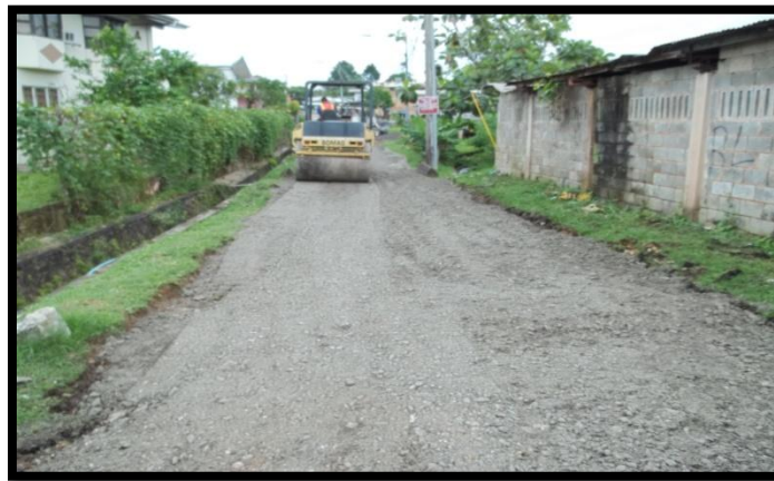
Picture 8: Showing compaction of base course material
