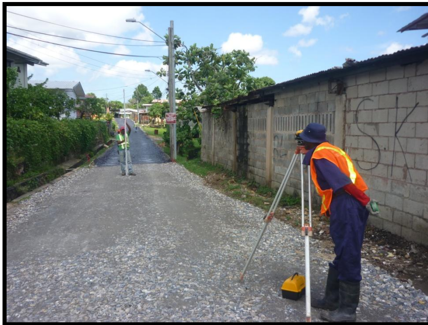
Picture 24: Showing surveying level – check levels for base course
