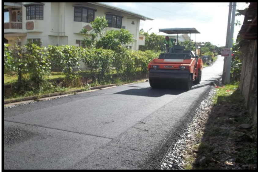
Picture 19: Showing primary compaction of asphaltic mix using oscillating roller
