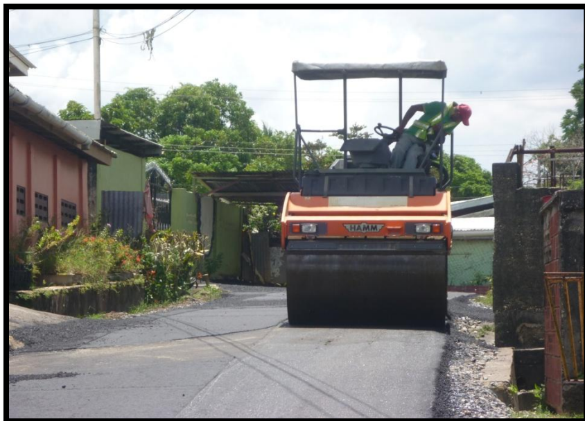
Picture 20: Showing primary compaction of asphaltic mix using oscillating roller
