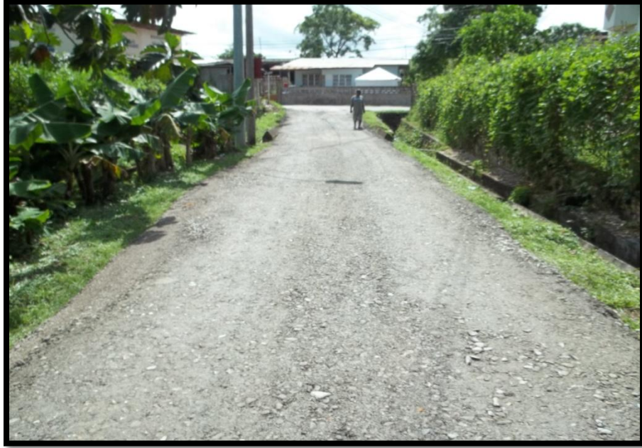
Picture 10: Showing compacted base course surface
