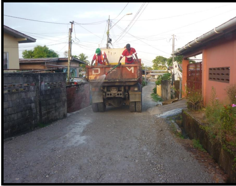
Picture 14: Showing water truck on site – for dust control
