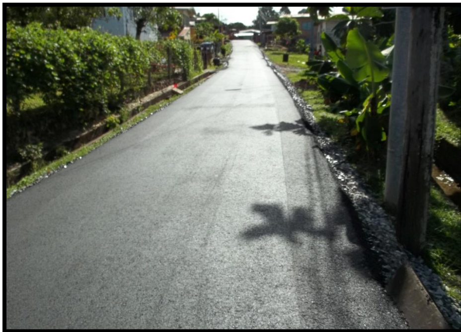
Picture 22: Showing final asphaltic wearing course
