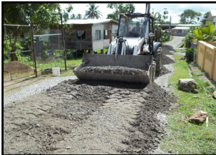
Picture 6: Showing use of backhoe to spread base course material
